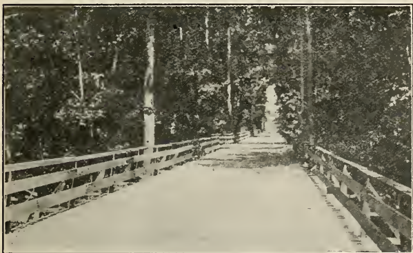
BRIDGE (900 FT.) ACROSS LAKE CHUMUCKLA.
